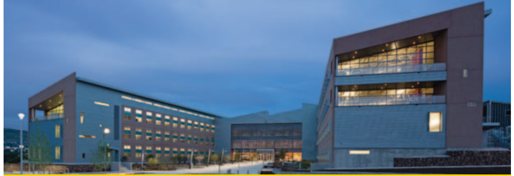
The RSF is expected to be the nation's largest ultra-efficient building. (Courtesy of Frank Ooms, Frank Ooms Photography)
